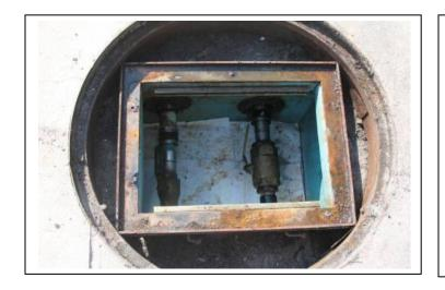
These two valves shut off the fuel supply from the tanks to the fuel dispensers. They are located in the ground near the water main and backflow valves. They should be in the off position when preparing for a hurricane.
