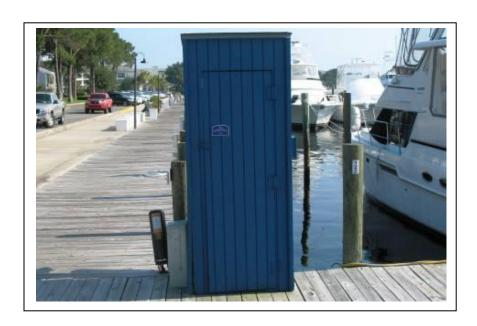
This electrical panel is located near slip 145. The main breaker in this panel should be in the off position when preparing for a hurricane.
