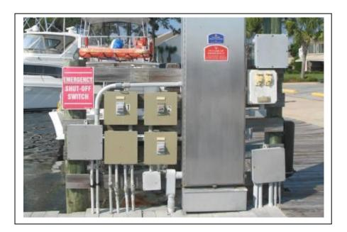
This electrical panel is located adjacent to the fuel shutoff switches at the entrance to the fuel dock. The main breaker in this panel should be in the off position when preparing for a hurricane.
