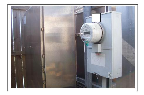
The large cabinet contains the breaker switches for Lift Pump, North and Middle Docks and the main switches to shut down the power to the main fuel tank's pumps.
