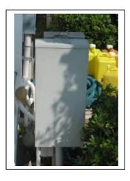
This is the Marina Office electrical shut off box, located on the south side of the building behind the pool pump box. This panel should be the last electrical item turned off when preparing for a hurricane.
