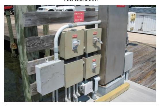
Pictured here are the fuel switches, located at the entrance to the fuel dock. The two upper switches (labeled 1 and 2) are for the diesel lines. The lower switch is for gasoline. These should be locked in the off position. The electrical panel to the right of these switches is where the main fuel breaker is located.
